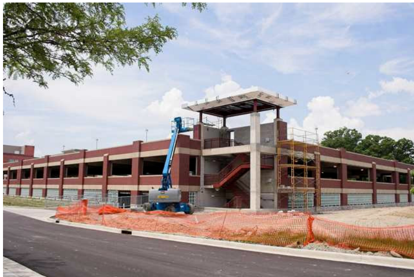
Lutheran Hospital, North Parking Garage
